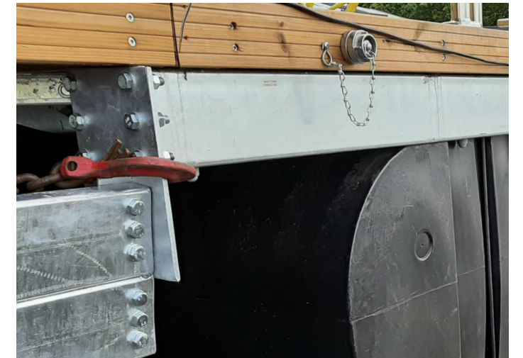
WASTE PUMP CONNECTION
